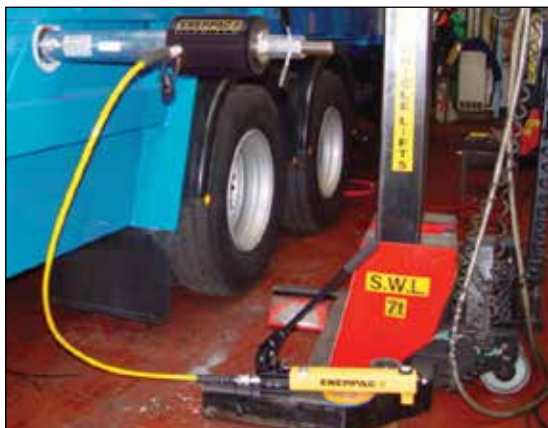
◀ An RACH306, powered by a P392 hand pump, is used to extract corroded carriage pins from refuse collection vehicles.
