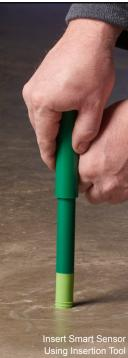
TIP: Check the L6 Smart Sensor prior to installation to ensure there is a properly functioning sensor that is giving a reading.
