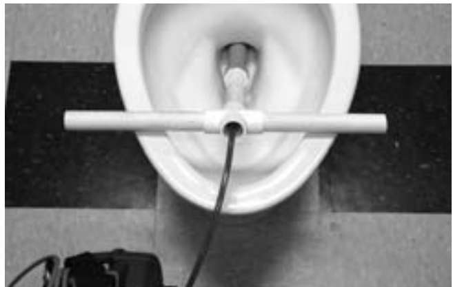
Figure 24 – Using A PVC Guide Tube
