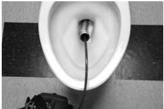
Figure 25 – Using The Flexible Guide Tube
