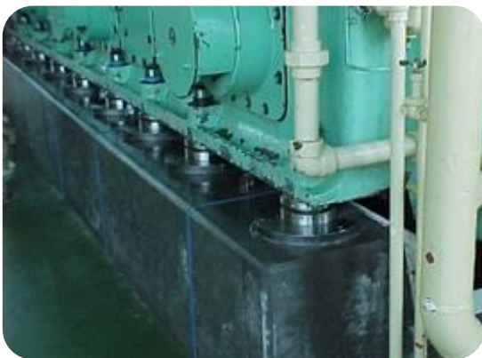
SKF Vibracon chock mounted on concrete with an additional steel plate to reduce surface pressure on the concrete.
