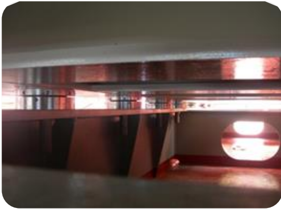
Compressor set chocked and mounted
