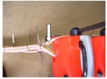
Outgoing and incoming legs are immediately brought back together and tied with tape, straps or bridles as they exit the raptor's hole, so that the 'air' between both is reduced to the minimum possible. The smaller this 'air' is, the less inductive impedance will be added.
