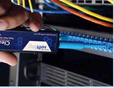
Remove cap for cleaning adapters and bulkheads
