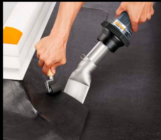
Overlap welding on a light dome.
