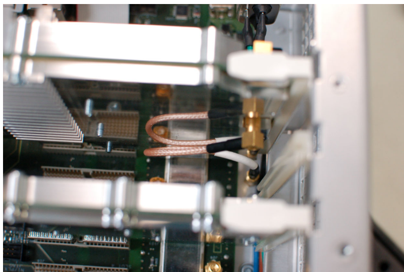
Figure 4: Reconnecting the cable on the back of the acquisition board
