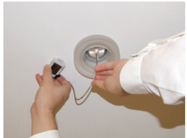
A fiber optic light pipe helps target a specific light source
