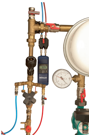
Fig. 3.1.2: Test hoses connected to fitting
