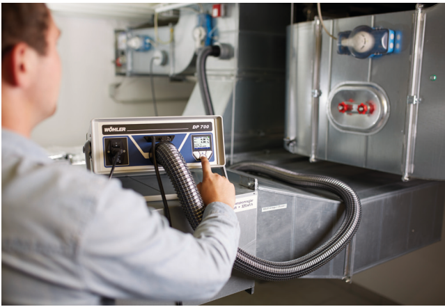
Leakage tests on several 100 m² of installed ductwork systems.
