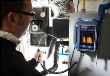
Fig. 45: Spillage test: Searching for condensate
