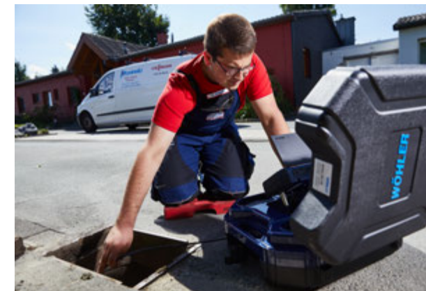
Secure drain inspection with the waterproof camera head.
