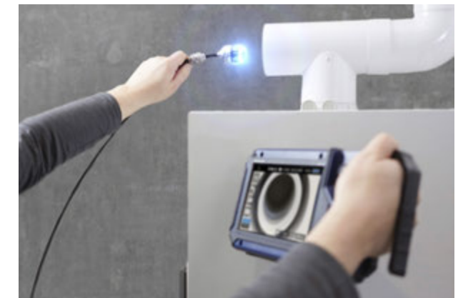
Inspection of flue gas lines from 2": easily negotiates tight bends of 87°.
