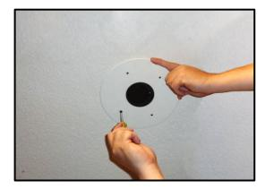
19) Install face-plate using Trim Mounting Screws (B).
