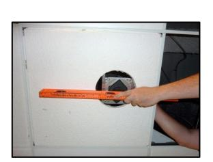
15) Using this anchor point, attach safety cable to building structure.(Safety cable not included)
