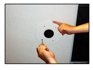
18) Install face-plate ring using Trim Mounting Screws (B).
