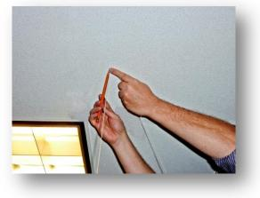
11) Be sure you have checked the clearances side to side and above the ceiling. Cut a 7  ${}^{3}/{}_{8}$ " diameter hole. The alignment ring may be used as a template.
