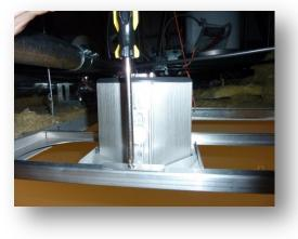
Note: If you need to change the orientation of the image to match the architectural specifications of the room, loosen the Mounting Tabs (C) and rotate the camera assembly as needed. Secure Tabs.
