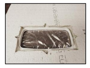
7) The tile must be notched on the center of all four sides to allow for the screw posts.
