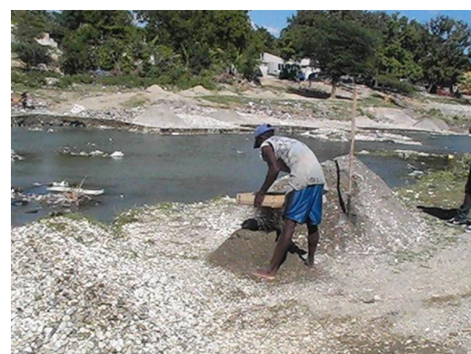
Riviera Grise experiencing artificial channelization as gravel and silt is manually removed.
