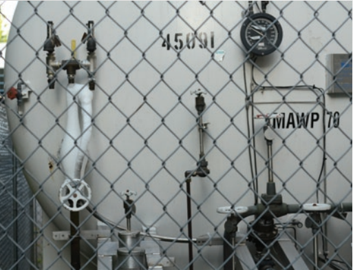
Difficult inspection sites
