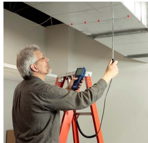
Duct traverse with Micromanometer and pitot tube
