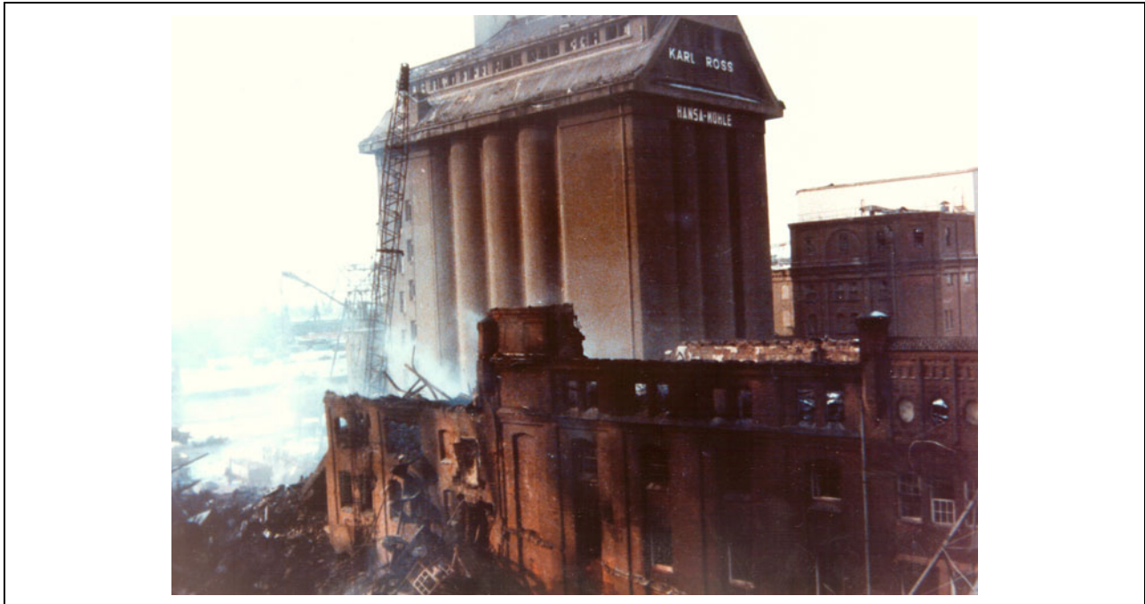
Figure 2: A mill after a dust explosion
