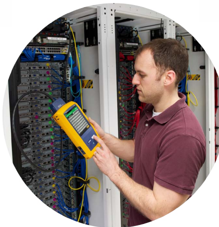
Network Engineers in Datacenters and Enterprise
