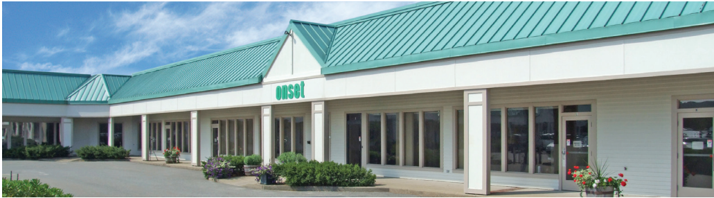
Onset headquarters, Cape Cod, MA
