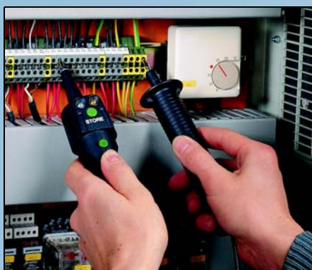
Protective conductor test
