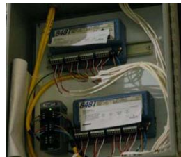
One 848T Wireless Temperature Transmitter can handle up to 4 inputs including 4-20mA, mV, Thermocouple, RTD, or ohm. The field hardened enclosure and intrinsically safe Power Module makes it ideal for this hazardous environment.
