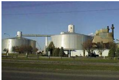
Sugar silos at ACS in EGF have a rotating bridge that made wired instrumentation impossible to implement.
