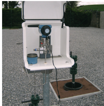
Rosemount wireless devices are placed in enclosures, standard practice for all instrumentation used at Bord Gáis’ AGIs.
