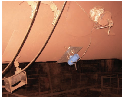
Rosemount 648 Wireless Temperature Transmitter connected to the kiln's existing thermocouples on a heat-proof ceramic seal.
