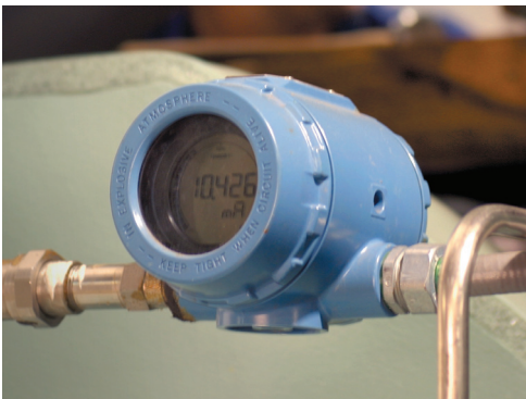
Figure 3.1.3.5b – Remote Mounted Field Transmitter
