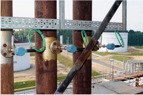
Figure 3.3.3.1a - Thermowell Installation Examples
