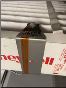
Sensor bracket installed on 2 inch filter.
