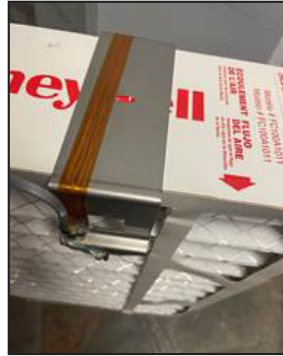
Sensor bracket installed on 4 inch filter.
