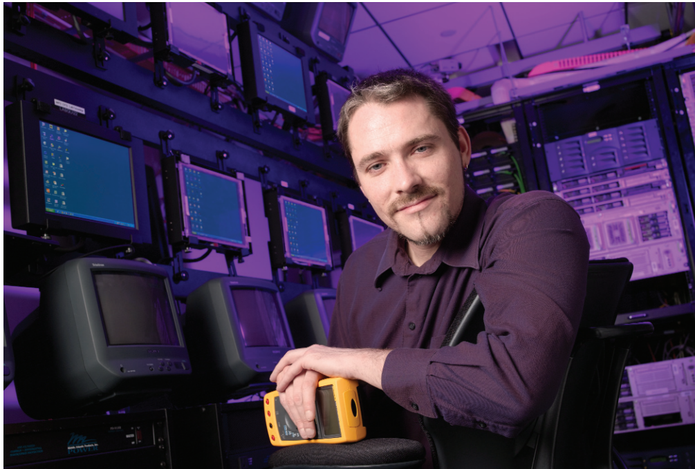
Grieshaber and his team custom-built this test rack to support software burn-in and performance testing for over 20 LCD touch panels, before installing the panels in the field. The touch panels are also a custom manufacture, and together with a PC they run proprietary Vulcan software for controlling A/V and environmental applications (from video to lighting).
