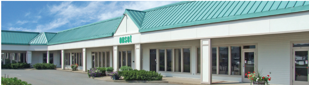
Onset headquarters, Cape Cod, MA
