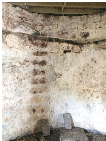
Figure 13: The fireplace Figure 14: The window from the interior Figure 15: The fixing holes for the ladder to the roof deck, with firing step above
