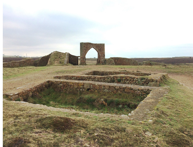
Figure 12: The gatehouse showing the drawbridge pit, portcullis groove and ditch beyond
