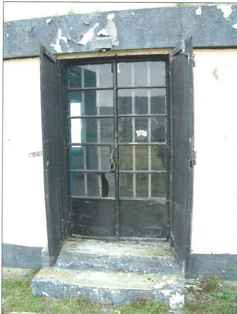
1930s metal window and doors
