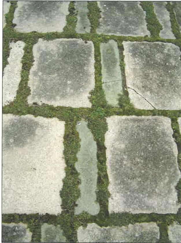
green and buff paving to platform
