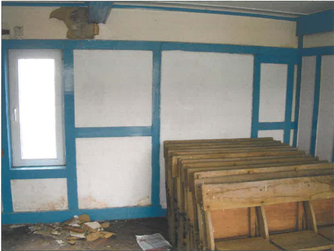
lounge looking west (with blocked doorway)
