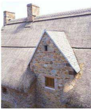
Hamptonne: restoration of the tourelle. A. The new gable and roof under construction. B. The completed tourelle, with a French slate roof and ceramic ridge tiles. Warwick Rodwell
