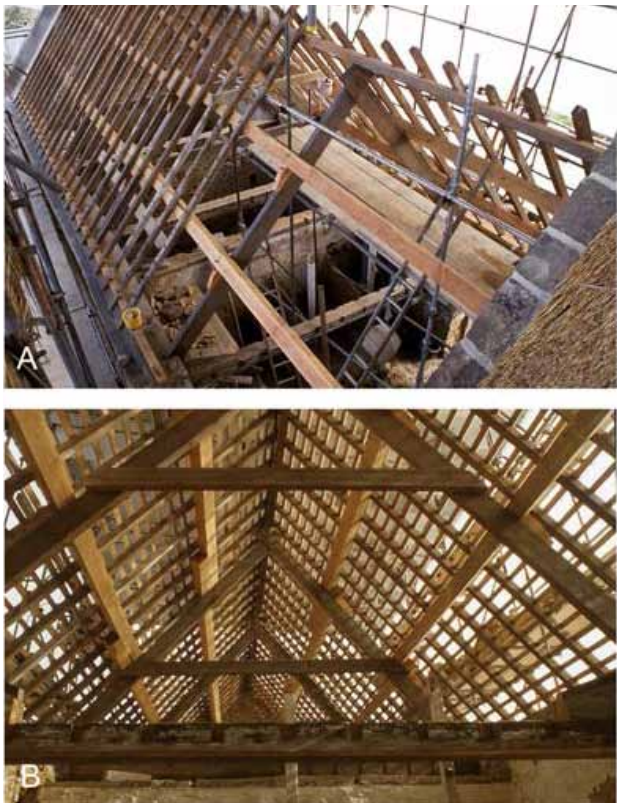
South Range. Construction of the new roof with A-frame trusses in progress, 1994. A. Exterior, looking south-east. B. Interior, looking east. Warwick Rodwell
