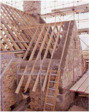
Hamptonne: restoration of the tourelle. A. The new gable and roof under construction. B. The completed tourelle, with a French slate roof and ceramic ridge tiles. Warwick Rodwell
