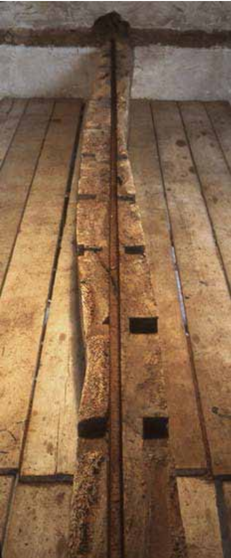
Hamptonne, east wing chamber. Slot cut to receive a stainless steel flitch plate in the upper face of the bridging-beam that supports the first floor. Warwick Rodwell Hamptonne, chamber. Terre battue floor under construction, 1992. View east. Warwick Rodwell
