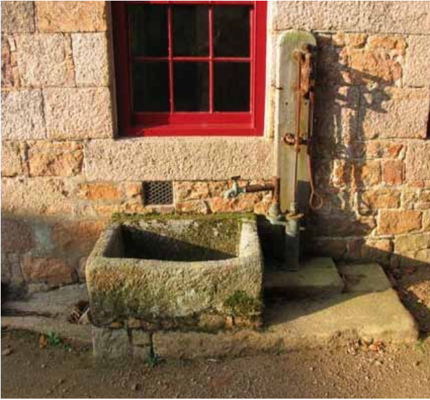
Syvret: east wall, exterior. Restored pump and cistern above the well. Warwick Rodwell
