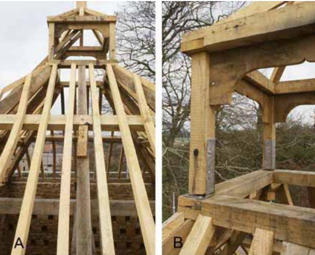
Dovecote: construction details of the roof and cupola. A. South side of roof. B. South-east corner of the cupola. Warwick Rodwell
