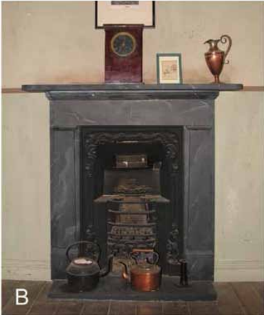
Syvret: chamber fireplaces. A. The timber surround painted to imitate Carrara marble. B. The timber surround painted to imitate veined black marble. Warwick Rodwell
