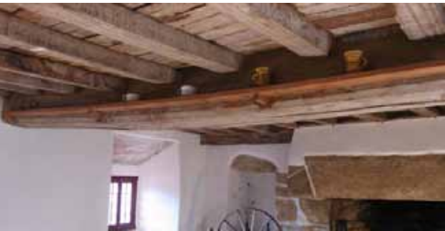
Langlois: hall. Note the reconstructed shelf supported by pegs on the side of a tie-beam which has interrupted chamfers. View south-west. Warwick Rodwell
