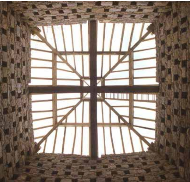
Dovecote: the skeleton of the new oak roof in situ on the dovecote, viewed from below. The structure is dominated by the two tie-beams which intersect at right-angles. Warwick Rodwell
