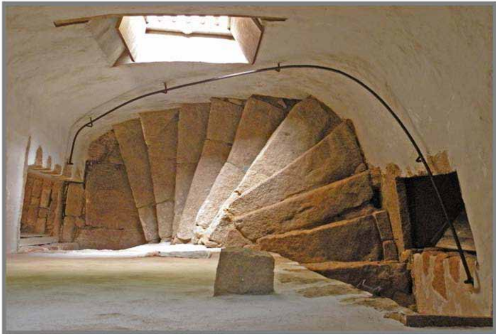
Hamptonne: the restored tourelle with the granite treads exposed. John Lord
