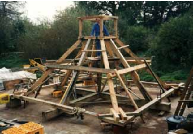
Dovecote: the new pyramidal roof frame under construction at ground level. Peter Huelin
