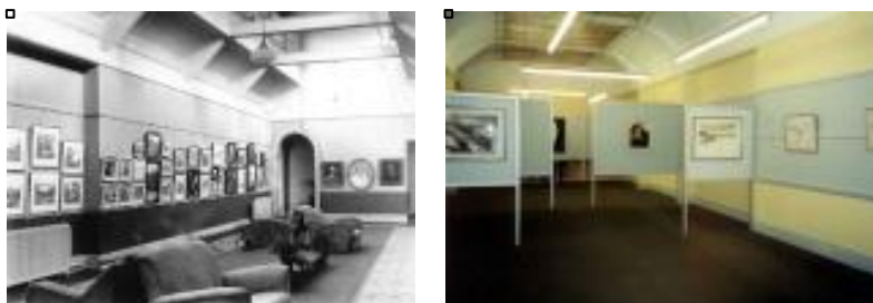
Figure 1.6 a The Barreau Art Gallery in 1940 (SJPA/010802) b and in 1988, shortly before it was demolished, photo by Geroge Drew (SJPA/011814)
