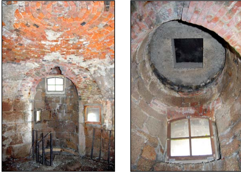
access to roof platform
