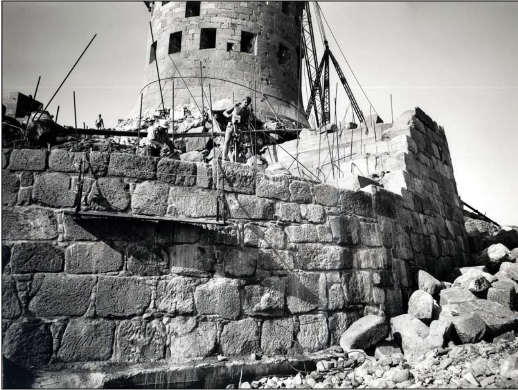
photograph of repair works underway
