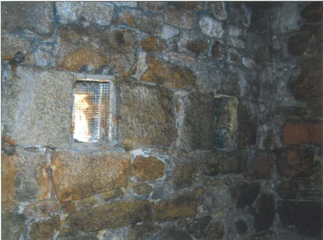
north wall showing gun embrasures overlooking doorways
