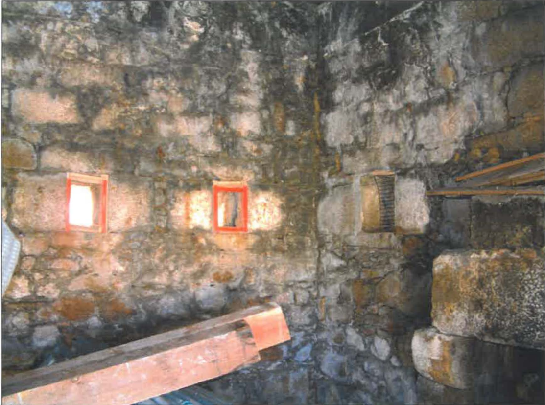
south and west walls showing gun embrasures
