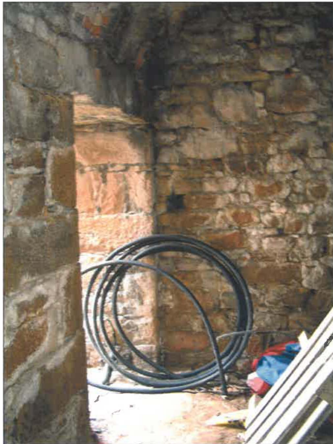
outer cell looking towards entrance door
