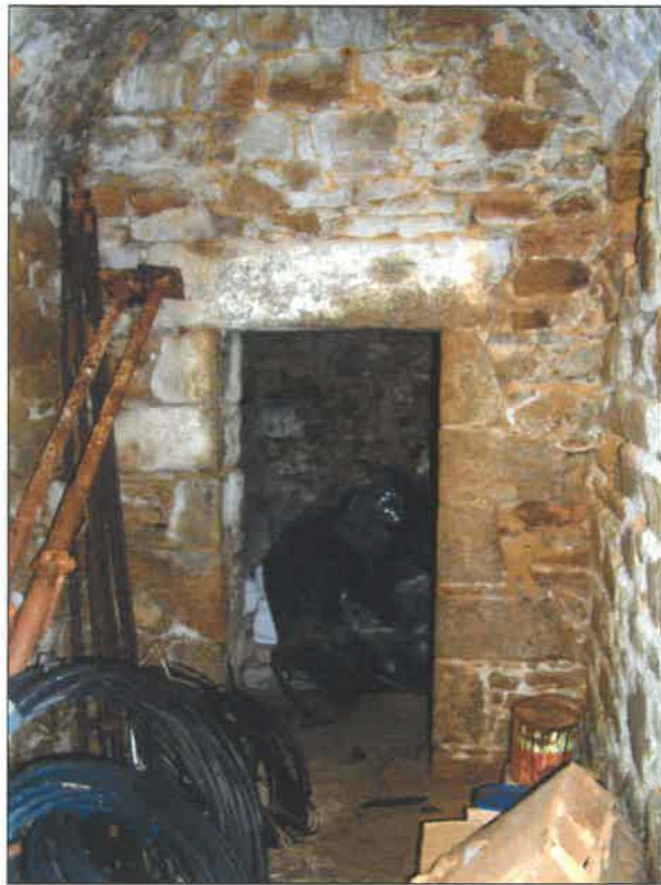
outer cell showing brick vault and door to inner cell
