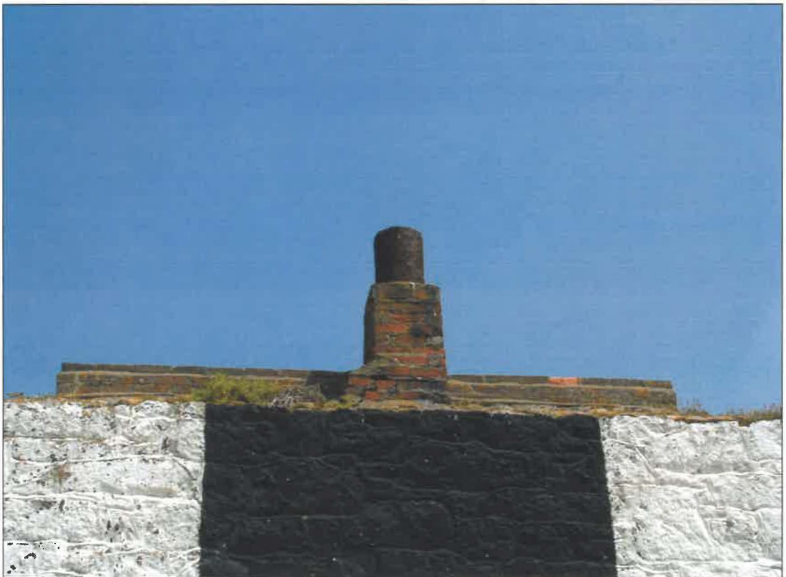
detail of roof and chimney
