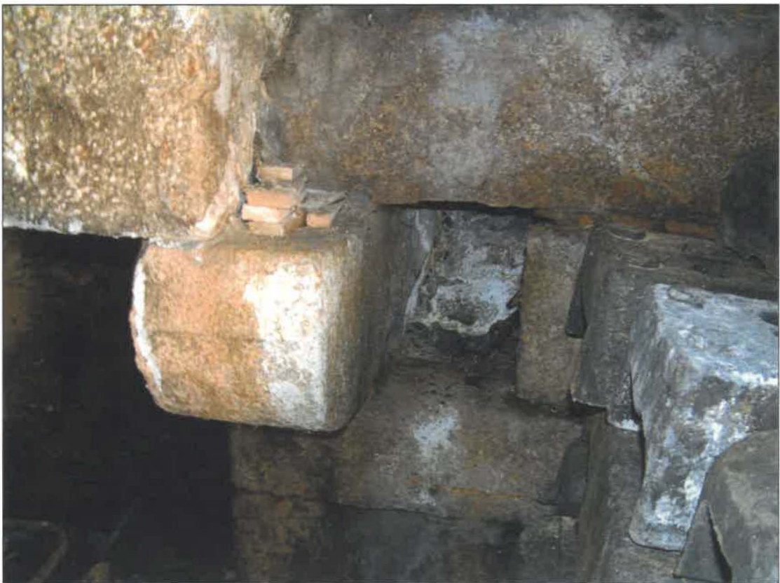
detail of corbelled fireplace
