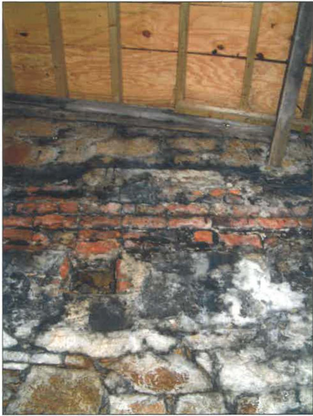
south and north walls showing beam sockets
