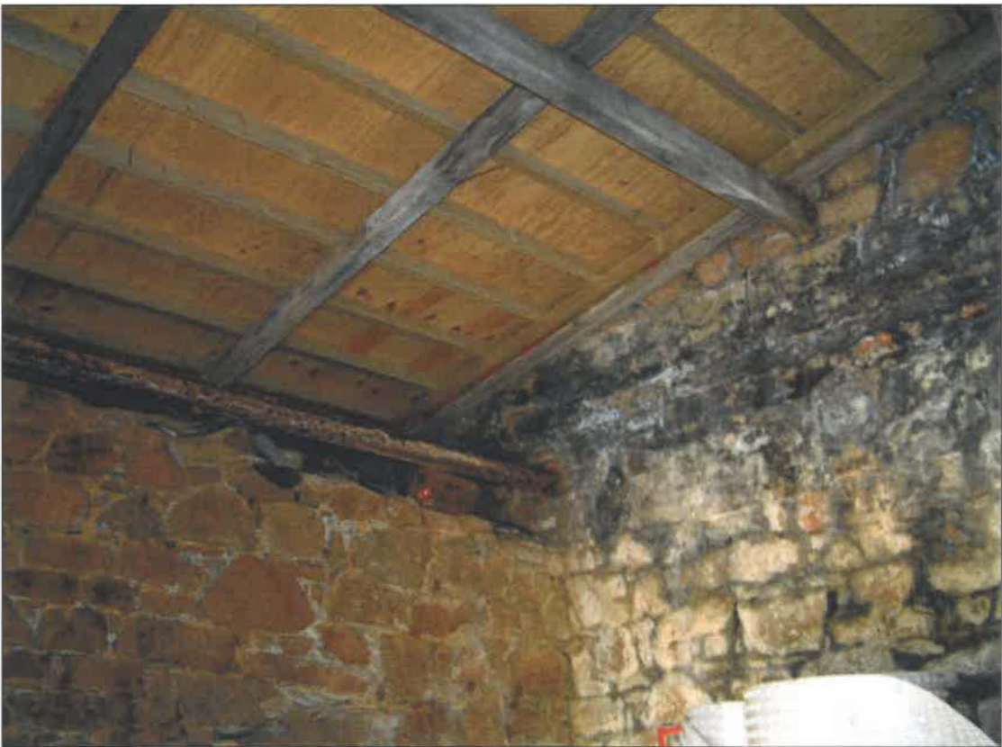
north-east and south-east corners
