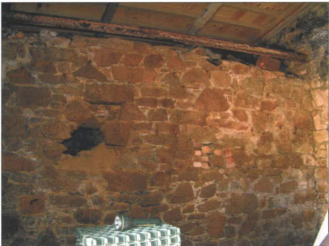
east wall separating the guardroom from the magazine
