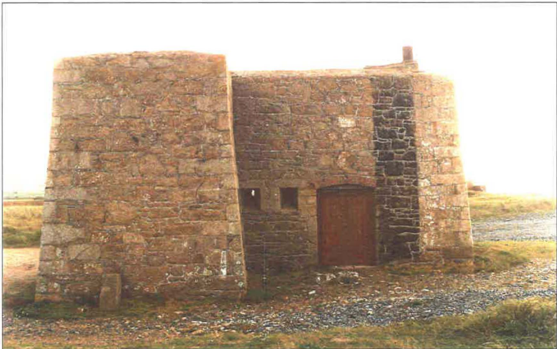
north elevation showing batter of walls
