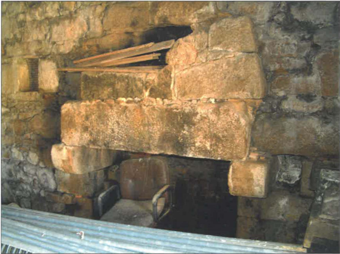
west wall showing corbelled fireplace and gun embrasure
