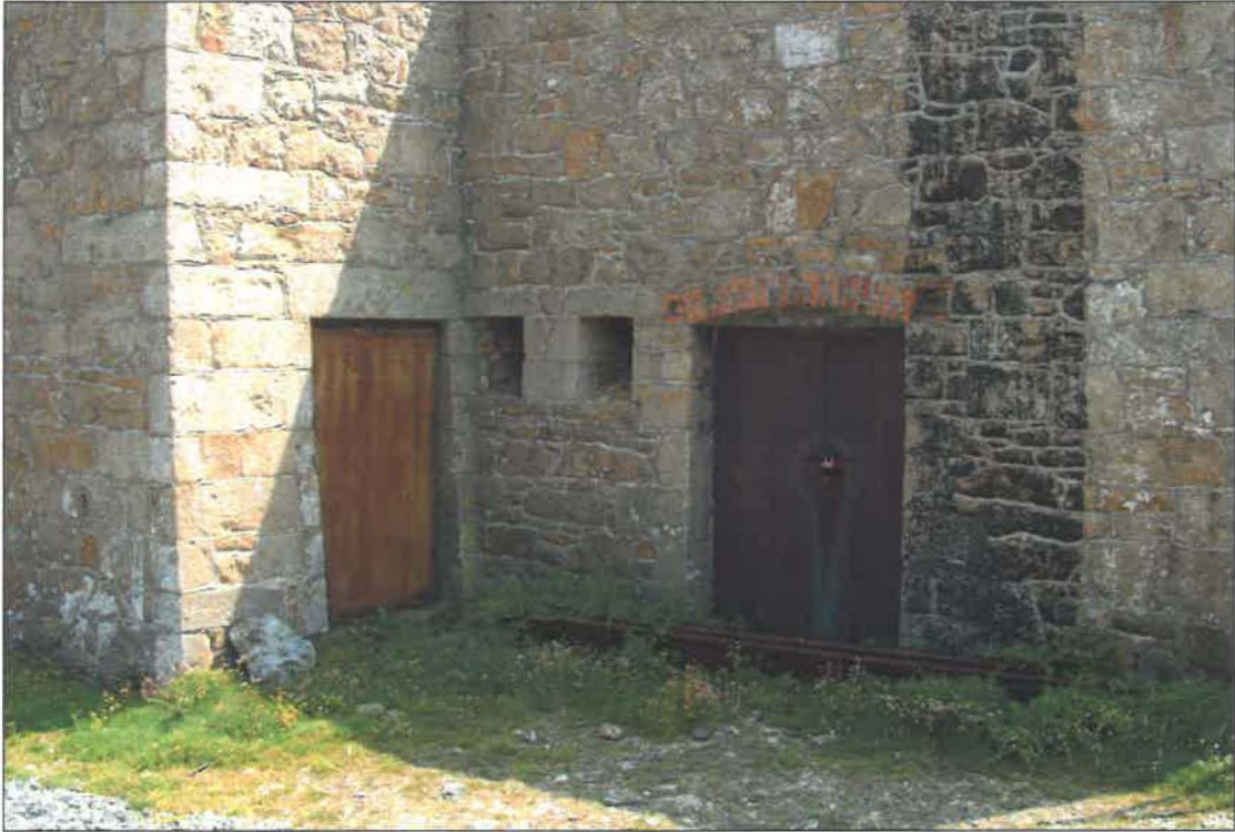
door into magazine (left) and door into guardroom (right)
