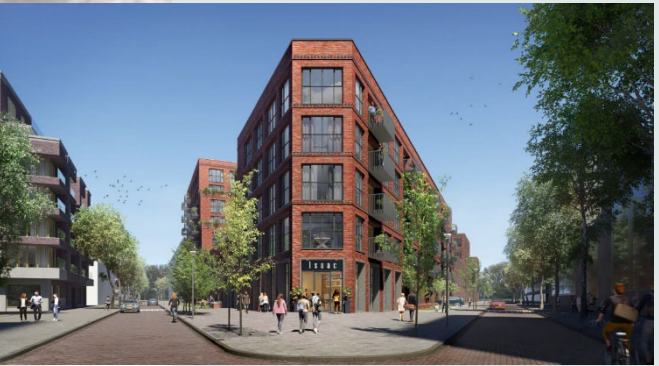
The Newton (residential): Under construction, delivery date in 2023.
