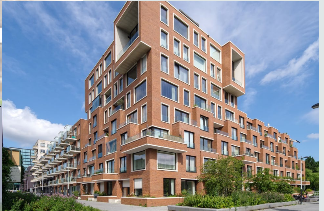
RIV (residential): finished
