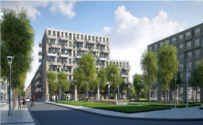
Square Amsterdam (residential): finished
