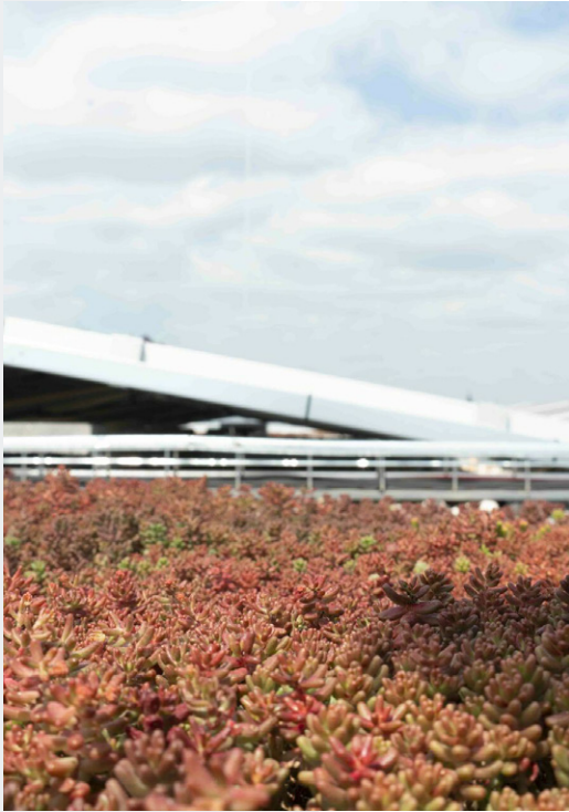
water retention roof
