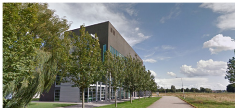
top: spinoza centre for neuroimaging bottom: building S
