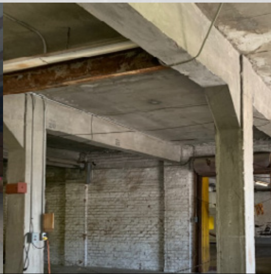
Building 5A Interior
