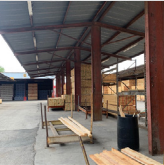
BLDG 14-17 Typical Interior
