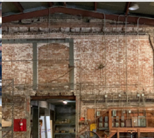
Bldg 6 Interior (Bldg 5A Adj. Brick Wall)
