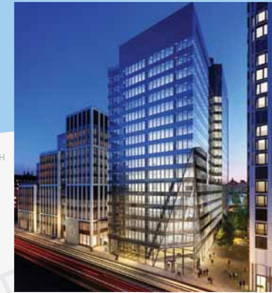
SOUTHBANK PLACE 1.5M SQ FT MIXED USE DEVELOPMENT CANARY WHARF / QATARI DIAR FULLY LET
