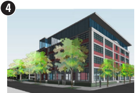
4 VOORHEES BUILDING 115,000 SF $35.00 PSF (FSG)
