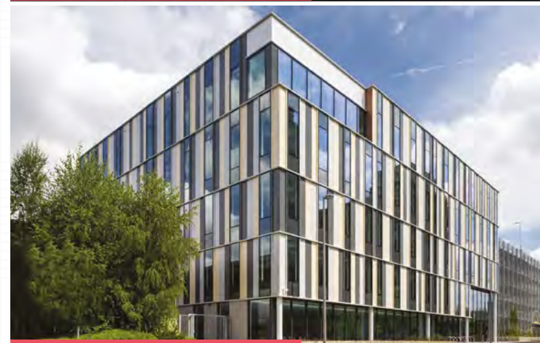
The Florence Building, Basingstoke
