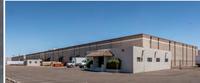
PHOENIX - SOUTH 35 DISTRIBUTION CENTER
