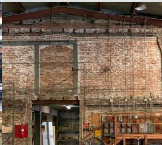
Bldg 6 Interior (Bldg 5A Adj. Brick Wall)
