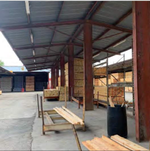
BLDG 14-17 Typical Interior
