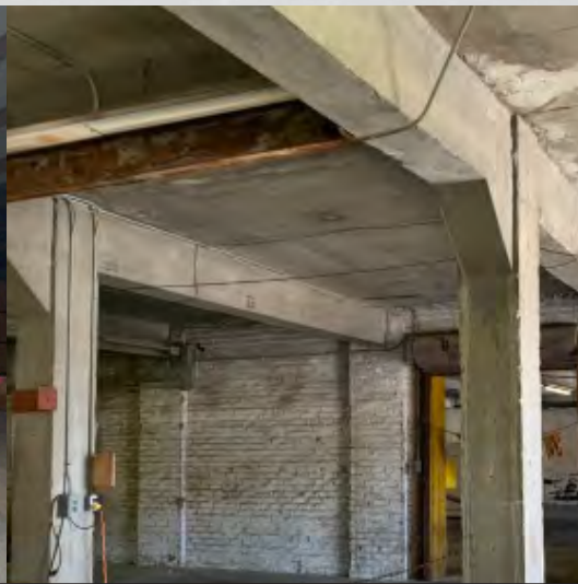
Building 5A Interior
