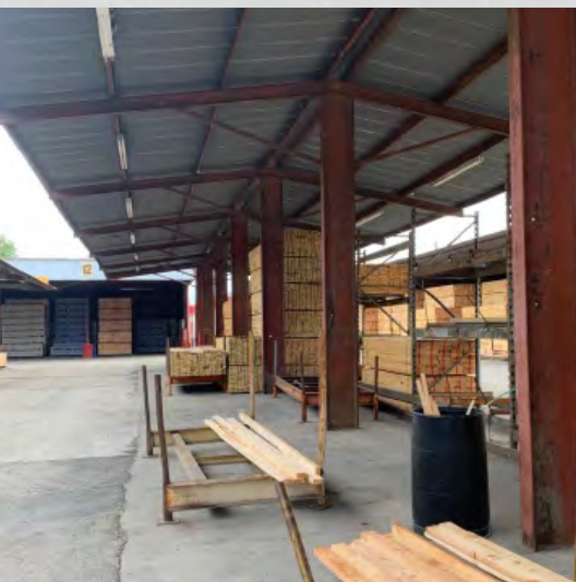
Bldg. 14-17 Typical Interior
