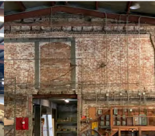
Bldg 6. Interior (Bldg. 5A Adj. Brick Wall)
