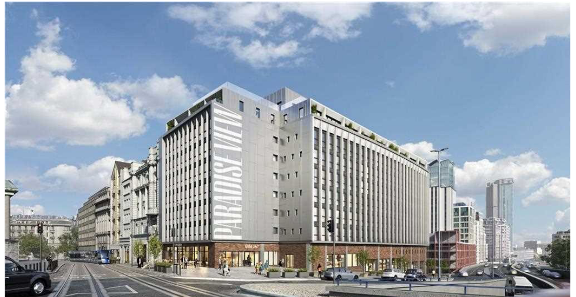
Paradise View – Under Construction
