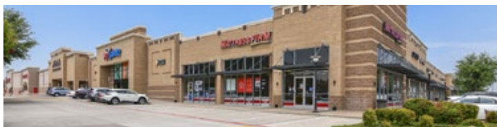
North Garland Crossing
