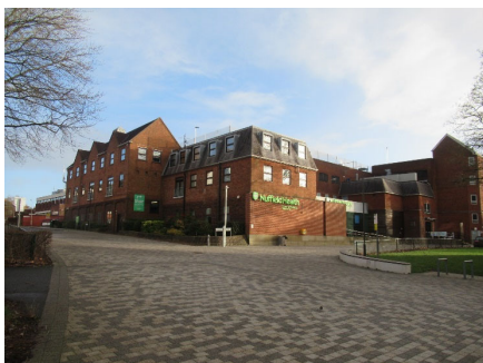
Photo of the front elevation.
