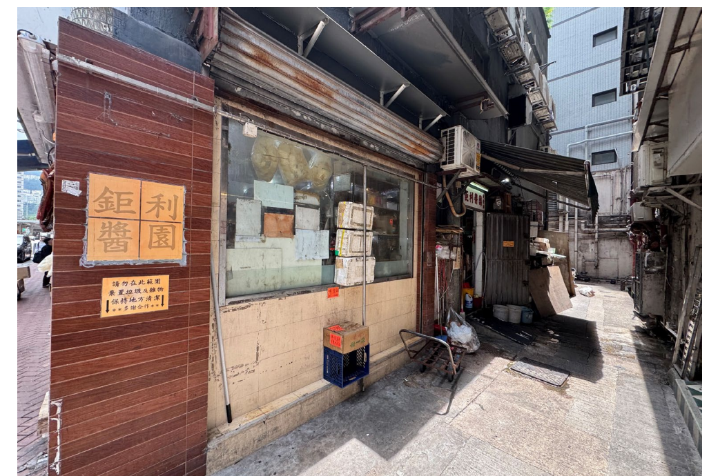
A舖之小巷門面 Frontage of Shop A facing the lane
