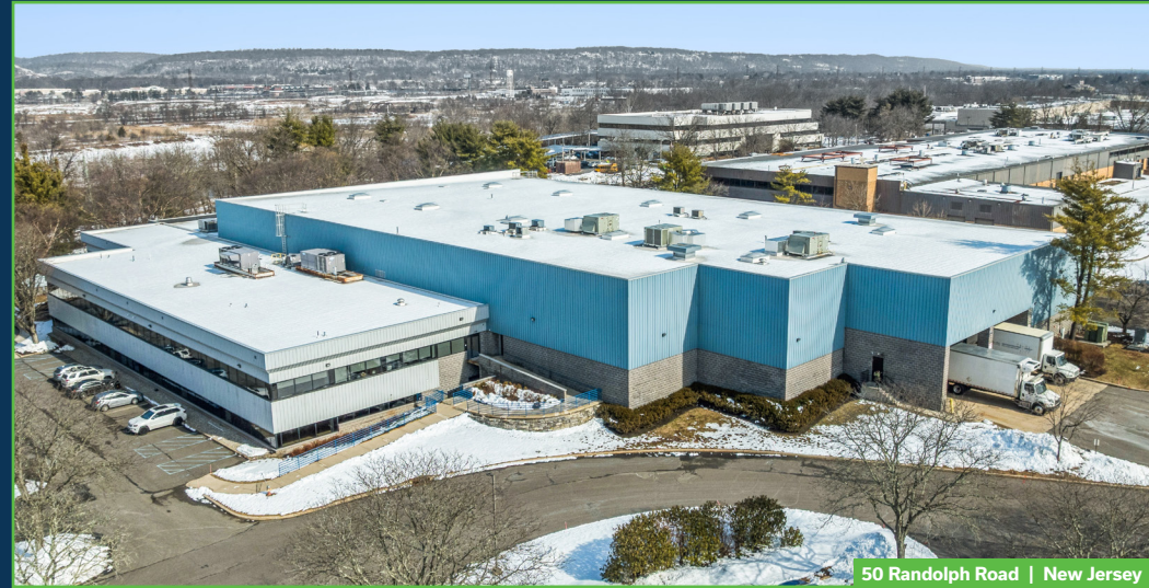
50 Randolph Road | New Jersey
