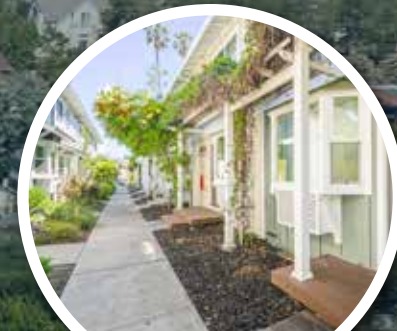
Landscaped Walkways with Grown-In Pergola Entries
