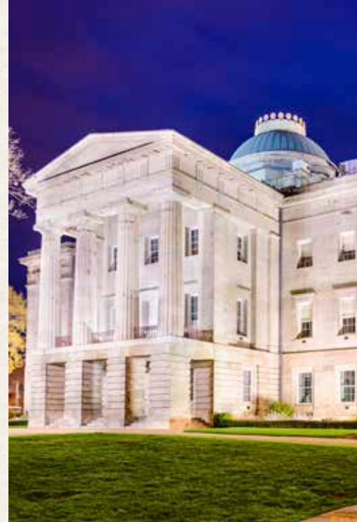
STATE CAPITOL BUILDING
