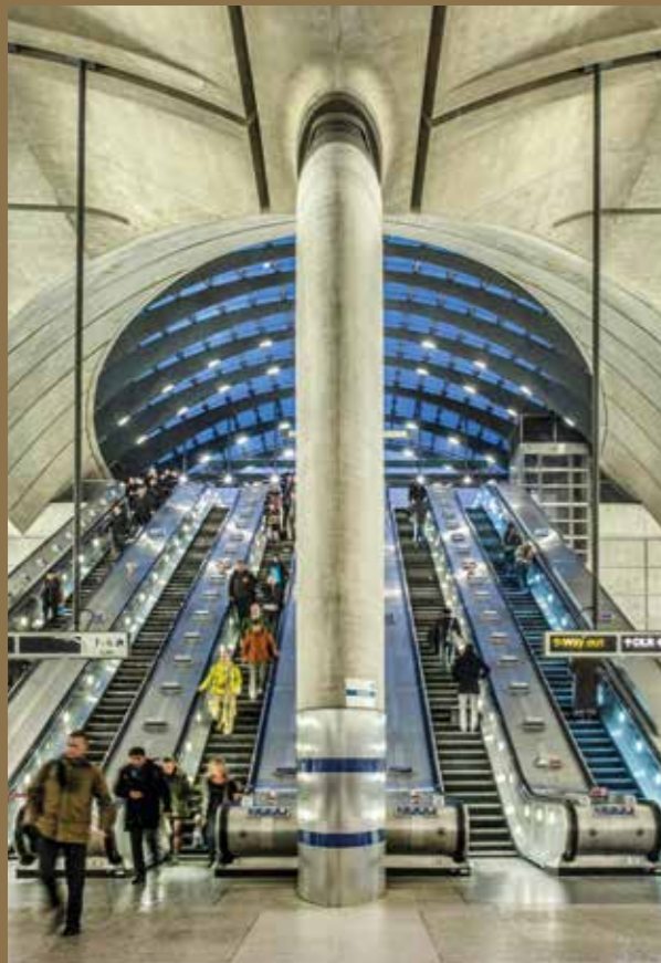
CANARY WHARF STATION
